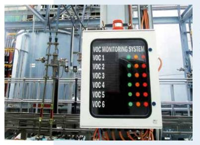
A real-time monitoring station in operation at Platinum's Precious Metals Refinery, indicating the current conditions for safe working in each area.
